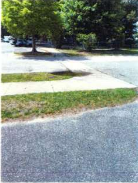
Crosswalk improvement/stripping from tennis court to playground.
